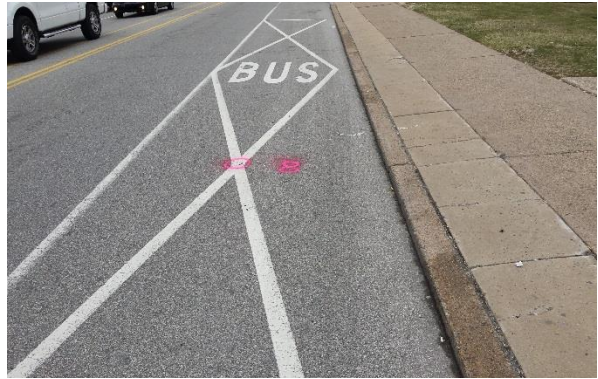
Figure 4: Typical detail of GCP
